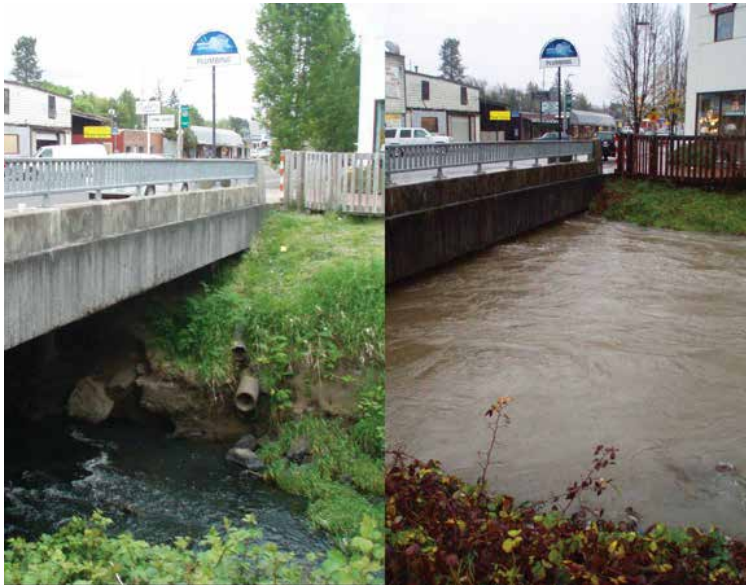
Impervious cover connected to storm drains causes urban creeks like Fanno Creek in Tigard to rise and fall rapidly.
