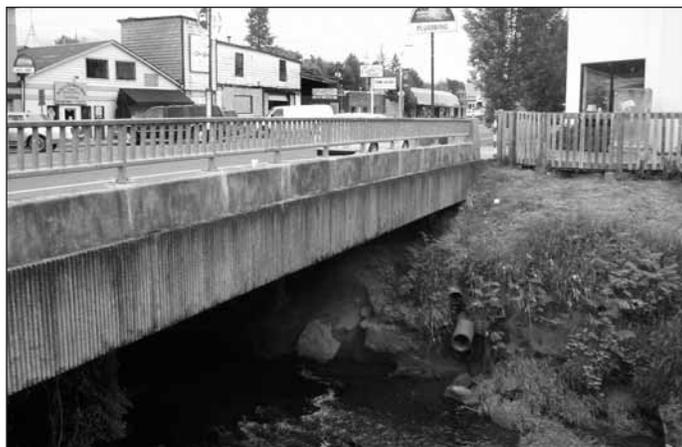
To convert Main Street into a green street, the City of Tigard will remove polluting drainage pipes that empty into Fanno Creek.
