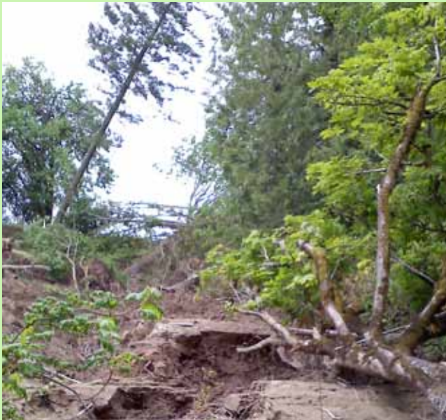
Erosion caused by poorly designed development.
